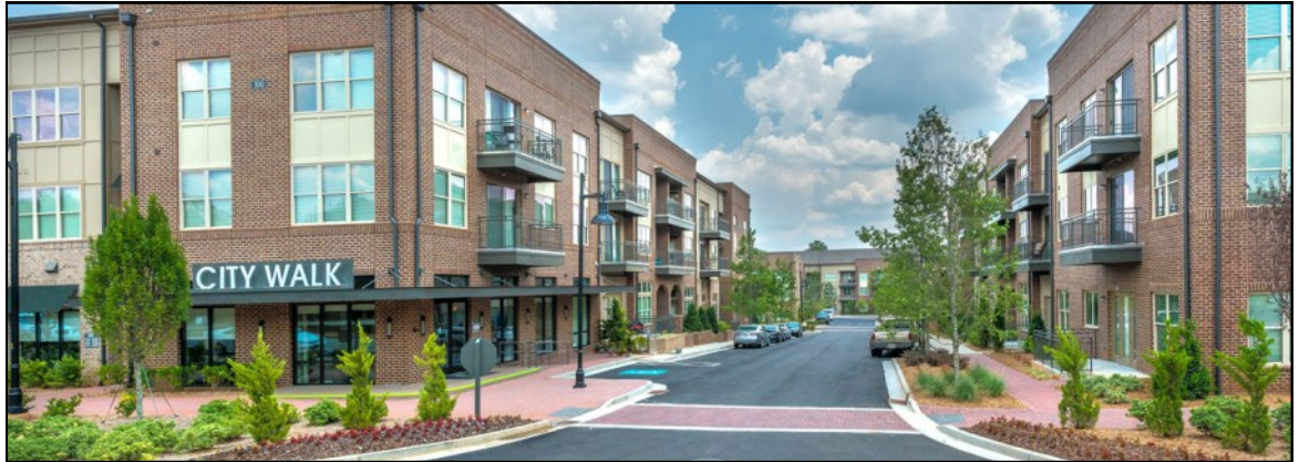
Completed City Walk Development
