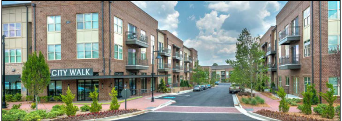
Completed City Walk Development
