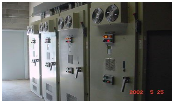
Current variable frequency drive equipment at plant
