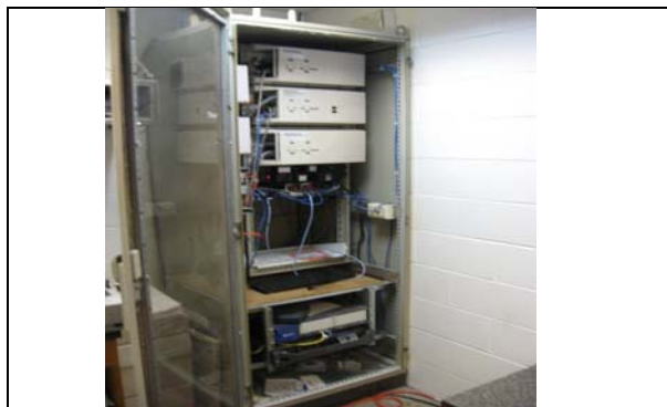
An existing SCADA unit in place at the I&D Water Plant.
