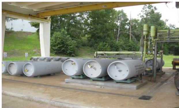
Chlorine tanks at the I & D Chlorine Building
