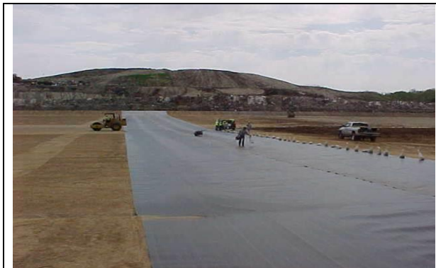
Early stages of new cell construction at landfill
