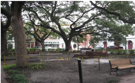
Repairs in Wright Square
