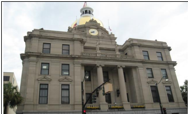
HVACs will be replaced in City-owned Facilities
