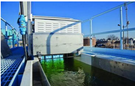
Discharged water passing through a UV disinfection station
