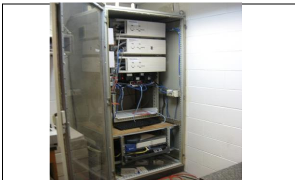
An existing SCADA unit in place at the I&amp;D Water Plant.
