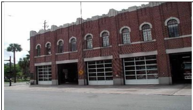
Fire Building Capital Maintenance
