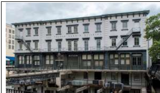
Gamble Building Capital Maintenance
