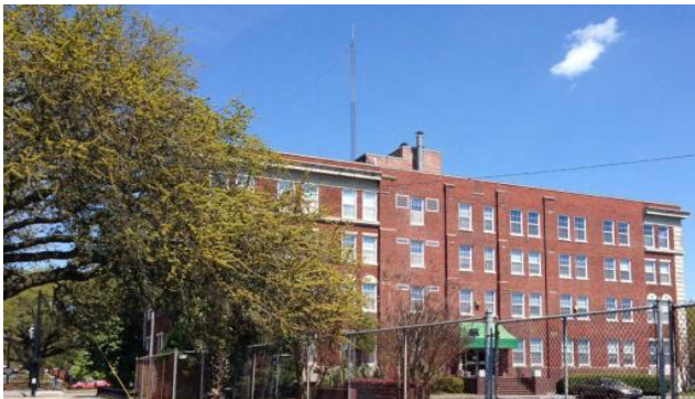
Liberty Municipal Building Renovations
