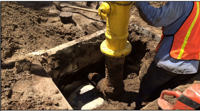
Fire Hydrant Replacement
