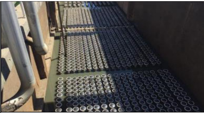
Zone 3 of 6 Diffusers in #1 Aeration Basin
