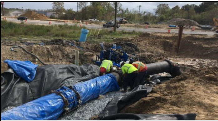
Installing a 24" Ductile Iron Water Main
