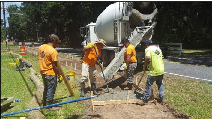
New Sidewalk Installation
