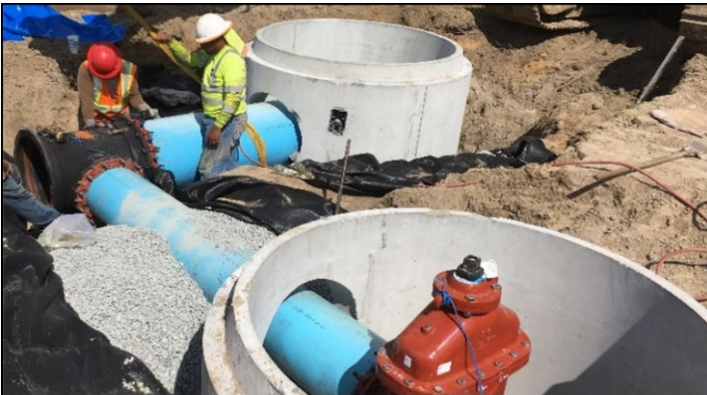
24" Water Main and Valve Installation
