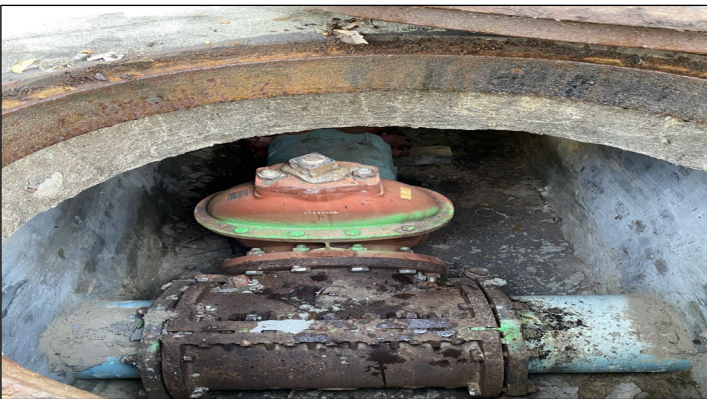
Pig Launching Structure at Lift Station 39
