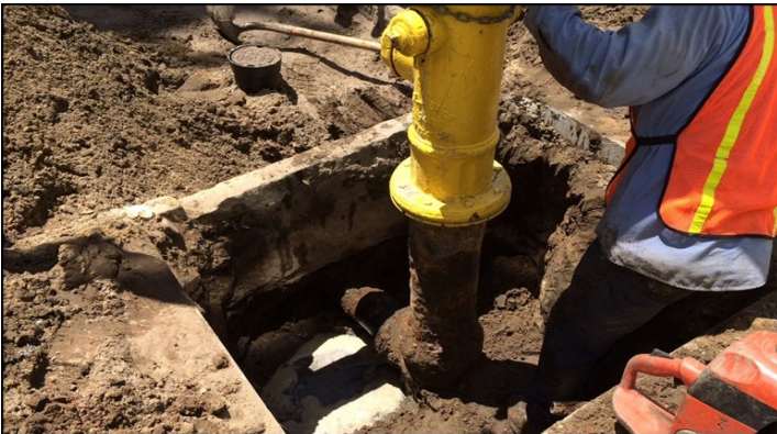
Fire Hydrant Replacement
