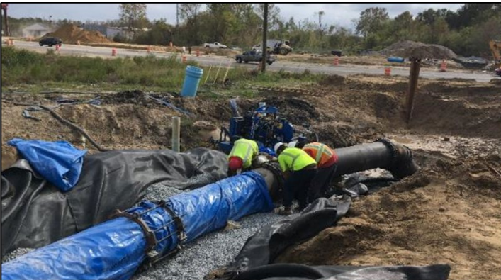
Installing a 24" Ductile Iron Water Main
