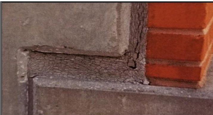
Failing Vertical Joint Sealant
