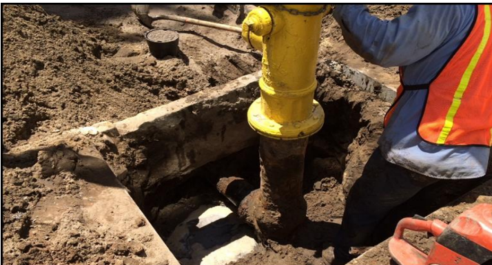
Fire Hydrant Replacement
