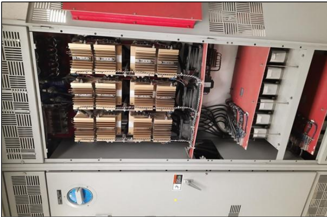
Variable Frequency Drive Cabinet
