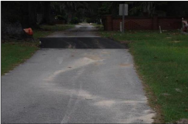
Asphalt Repairs in Laurel Grove South Cemetery
