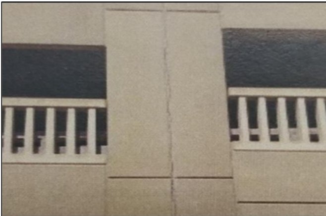
Precast Façade Sealant
