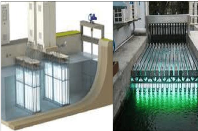
UV Disinfecting System Web Picture
