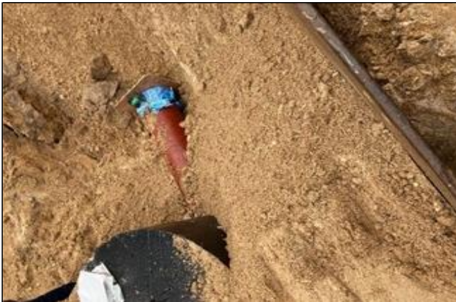
Coated Ductile Iron Pipe & Manhole 16" Force Main Installation
