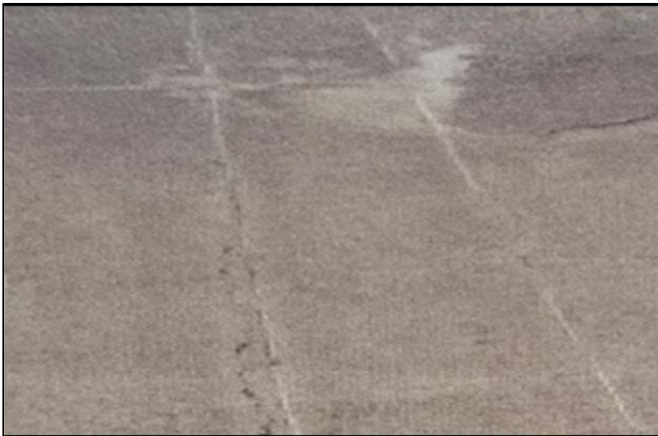
Existing Joint Sealant
