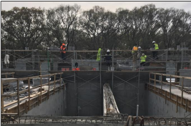
Membrane Tanks and Control Building Construction
