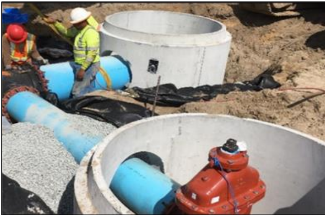
24" Water Main and Valve Installation
