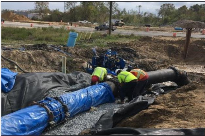
Installing a 24" Ductile Iron Water Main
