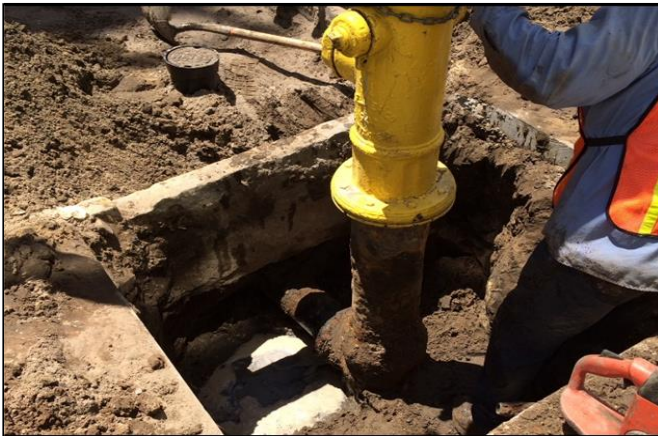
Fire Hydrant Replacement
