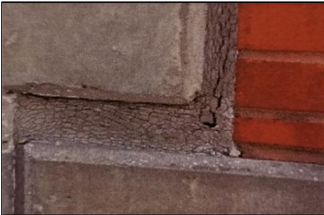
Failing Vertical Joint Sealant
