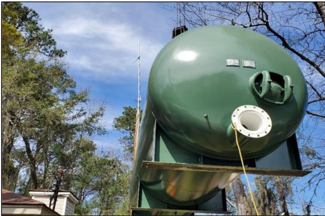
Installing New Tank at Well 28
