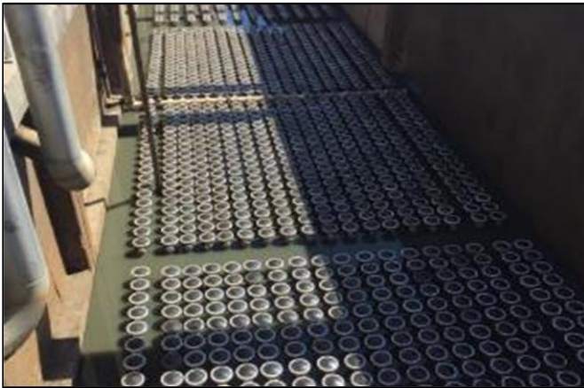
Zone 3 of 6 Diffusers in #1 Aeration Basin
