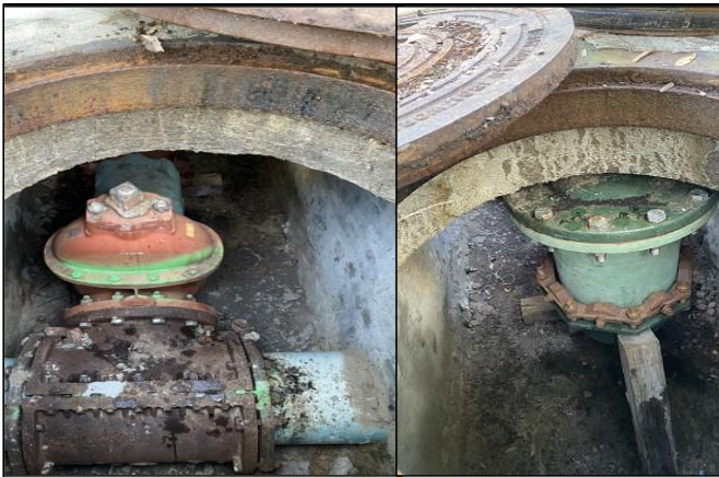
Pig Launching Structure At lift Station 39
