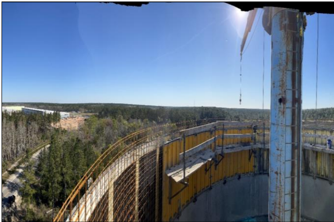
Typical Elevated Tank Construction
