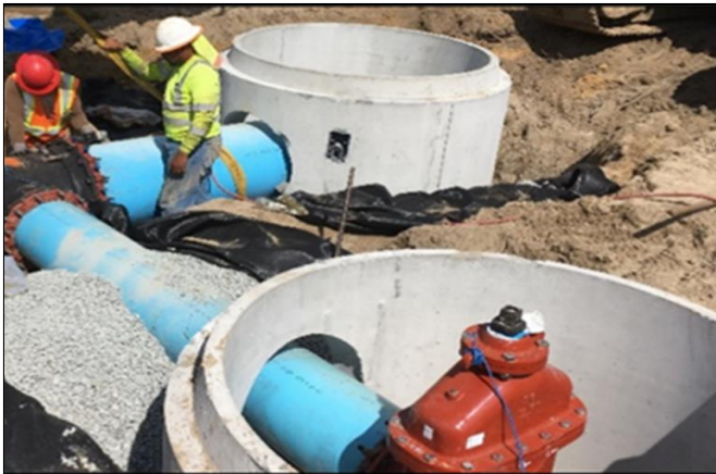
24" Water Main and Valve Installation
