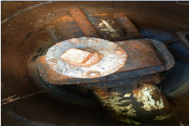
Typical Gate Valve in Manhole
