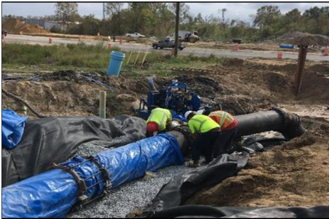
Installing a 24" Ductile Iron Water Main
