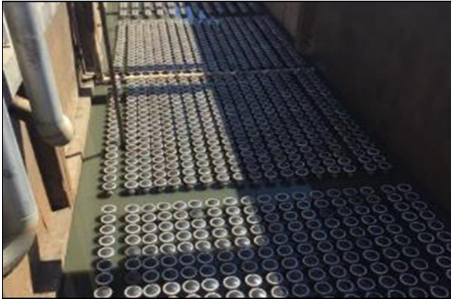
Zone 3 of 6 Diffusers in #1 Aeration Basin
