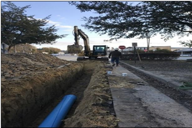
Typical 12" Water Main - Open Trench
