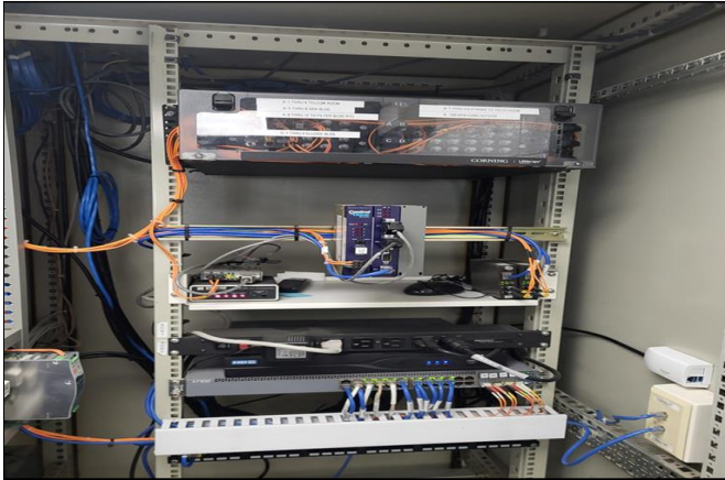
SCADA Controls
