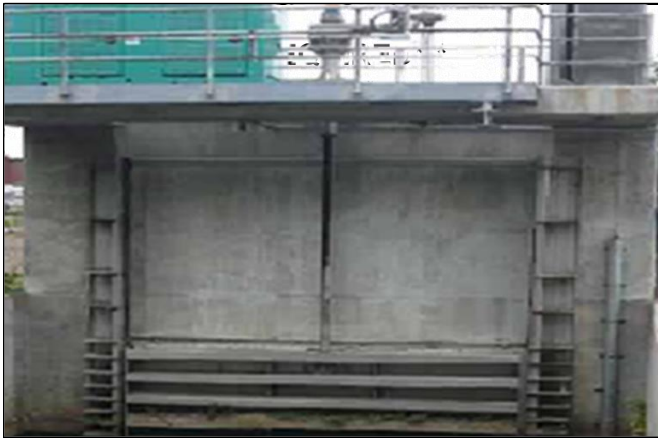
Sluice Gate
