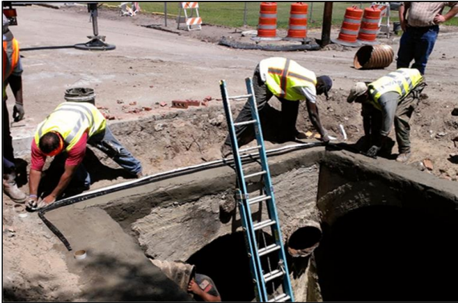
Storm Drainage Junction Box Repair
