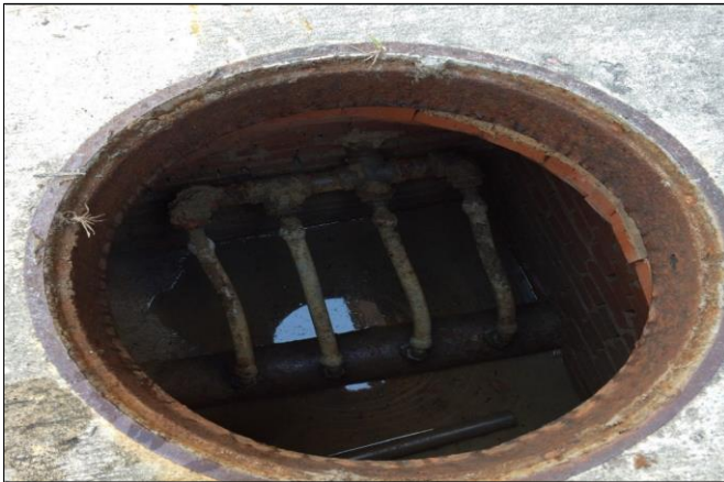
Water Service Gooseneck Connections to Main
