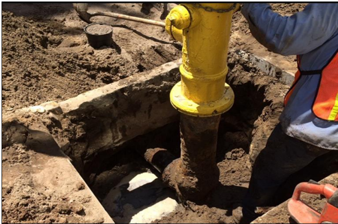
Fire Hydrant Replacement
