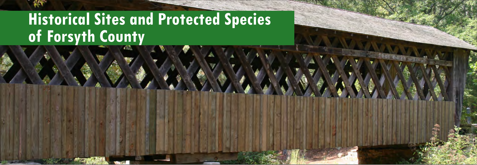
Poole's Mill Bridge
