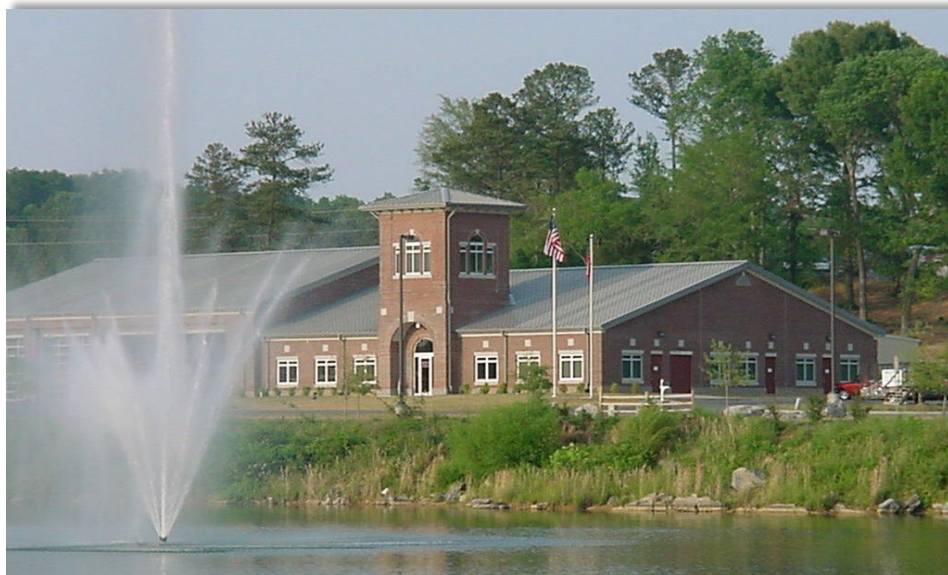
Gordon County Fire Station 1
