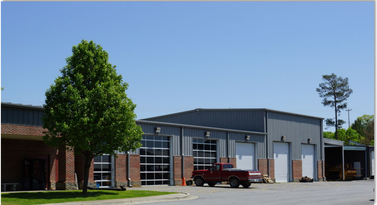
Gordon County Fleet Management Facility
