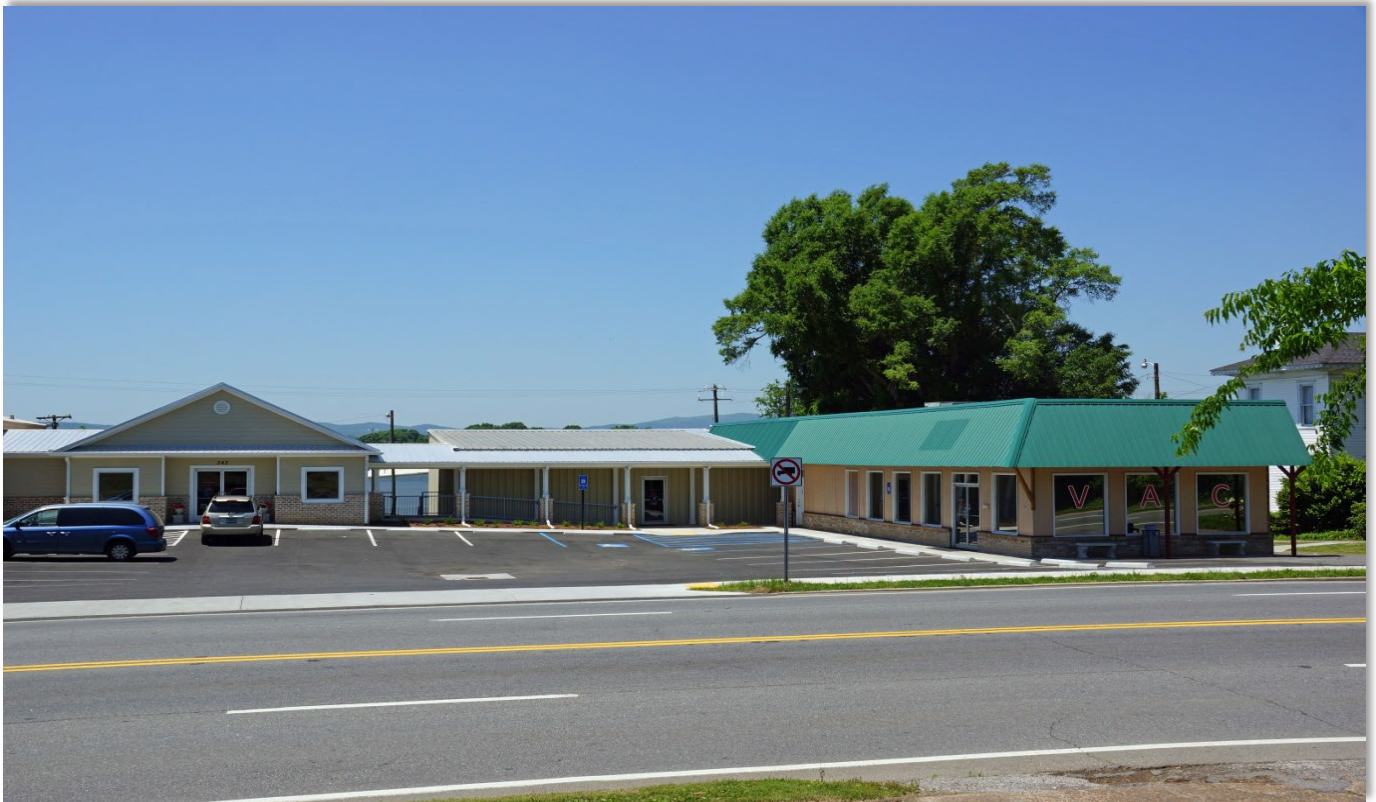
Voluntary Action Center Improvements
