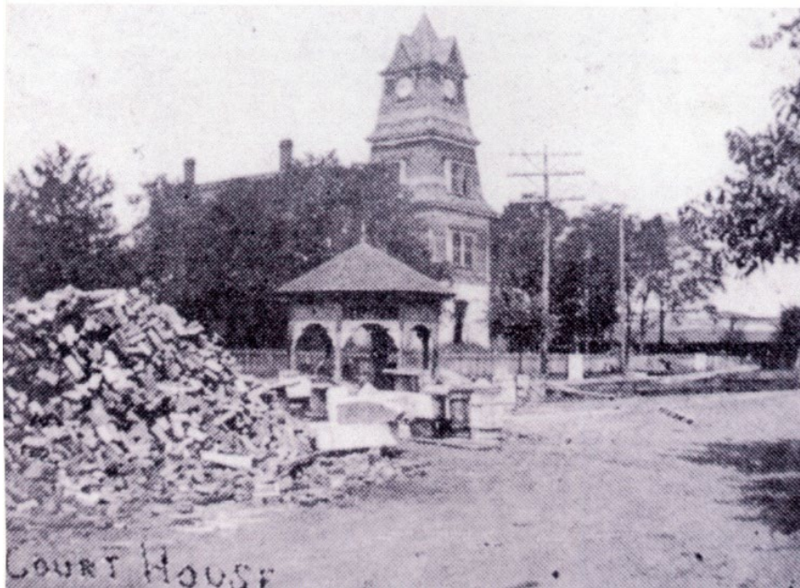
Courthouse of 1852. Note one of the corner wells in foreground.
