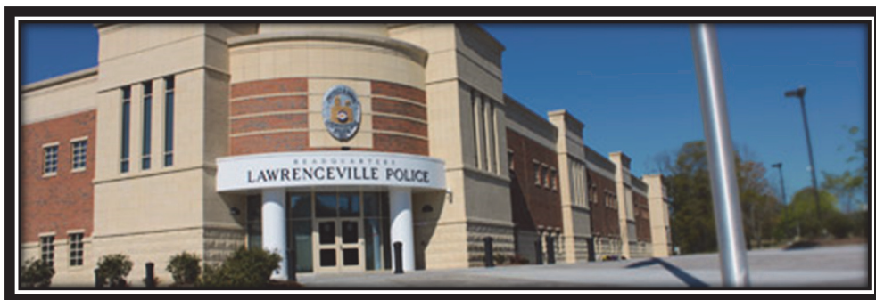
Lawrenceville Police Department Constructed Using 2005 SPLOST Funds
